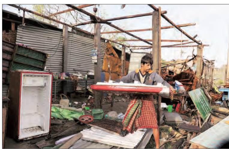
A heavily damaged shop in Bakkhali, South 24 Parganas
